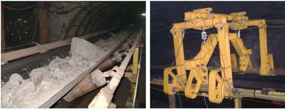
Figure 8. View of the conveyor and the assembled measuring unit.
