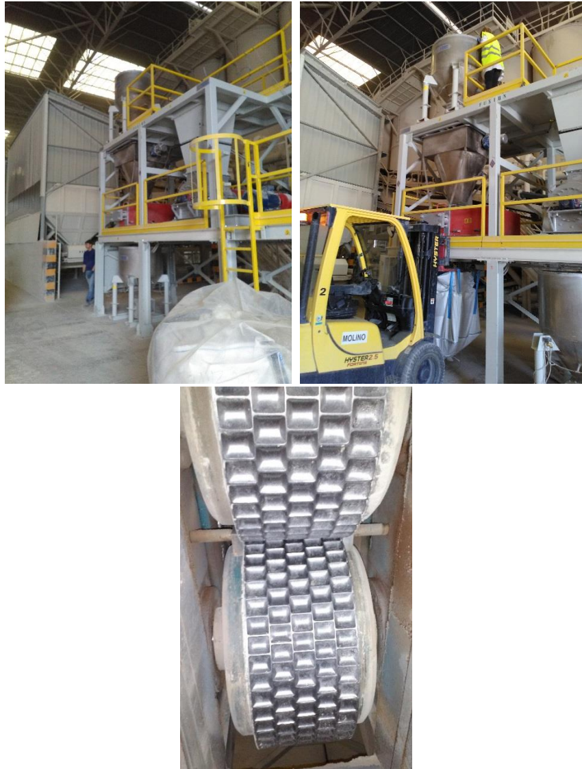
Figure 5. Pictures of the rolling-compaction pilot facility.
